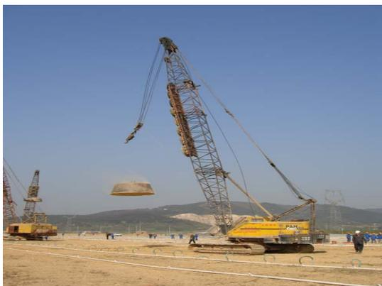
Fig 2.5 Dynamic compaction
