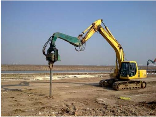
Fig 2.2 Vacuum pipe installation by hydraumatic method
