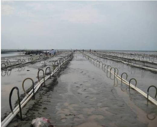
Fig 2.3 vacuum drainage system layout
