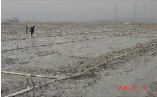
Figure 2. Array of vacuum pips and horizontal drainage pips.
