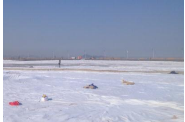
c) Non-woven geotextile installation.
