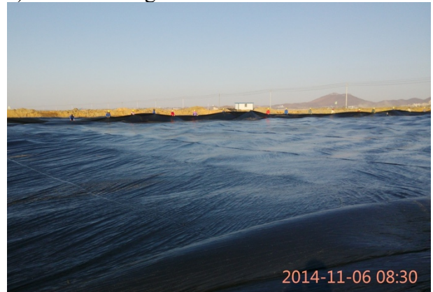
d) Geomembrane installation.
