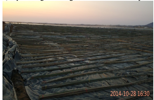
b) Installing bamboo grid.
