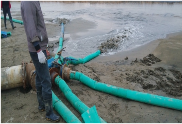
d) Backfill 0.4 m thickness sand by hydraulic filling method.
