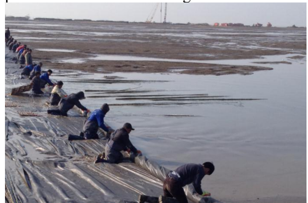
a) Spreading woven geotextile above slurry.
