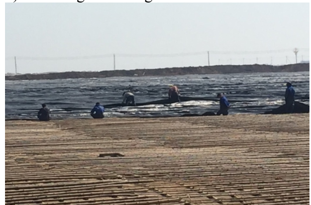
c) Spreading another layer geotextile above bamboo grid.
