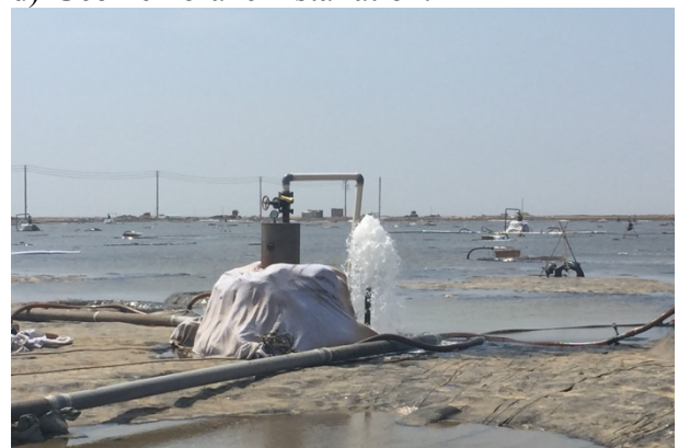
e) Vacuum pumps installation & running.
